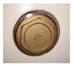
Place a suitable supplied gasket around the heater base. Keeping the heater element horizontal and square with the boss, insert the heater into the opening. Secure by turning the heater onto the threads.
