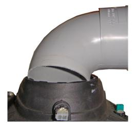
• Remove the flue elbow by twisting the flue elbow whilst lifting it up and away from the heat exchanger.
