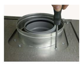
The appliance can be installed using a number of alternative arrangements depending upon the installation requirements It is delivered with a 130/200mm concentric outlet in the centre. Flue components are ordered separately as required.
