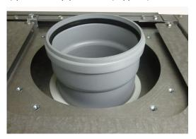
Screw metal air colar onto the top of the flue socket with the 8 screws (supplied) (see below)
