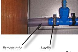
Release heat exchanger connections
