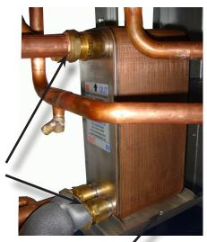
Remove screws from either side of plate heat exchanger
