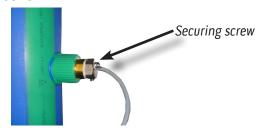
The LLH sensor is fitted into the top of the LLH in the rear top left hand side of the appliance.
