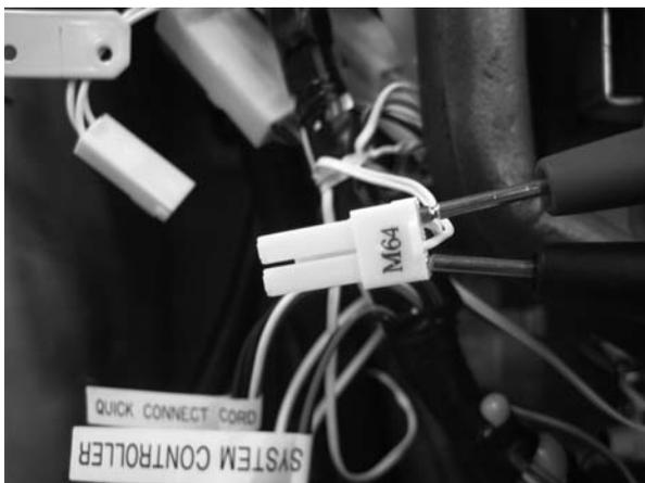
Check the water outlet thermistor.
