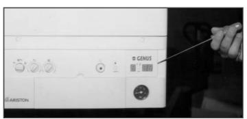
In the event of the chosen curve not being the most suitable for the type of system, it may be changed (selecting a more appropriate one) or moved until the desired thermal behaviour is obtained for the boiler and the system.
