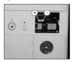
**NB:** The last effect achieved by adjusting the thermal curves is to change the behaviour of the system in relation to the room temperature. If the curve used has been selected underestimating the thermal needs of the building, i.e. it is too "low", it is possible that the building will not heat up sufficiently (the boiler will arrive to the set-point before the building reaches the desired temperature); the result is that the building will feel cold.
