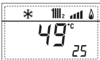
26. Visualisation safety thermostat with board ZONA MIX 2 (input S1) respectively ON and OFF
